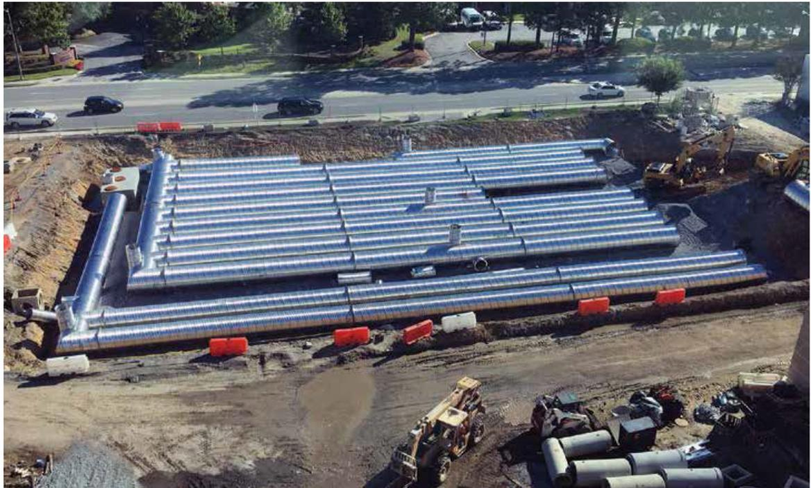
For the majority of applications, corrugated metal pipe (CMP) is the "go to" material for stormwater detention and infiltration. With its low cost, a wide variety of diameters, layout configurations and coatings, no other material can match CMP's flexibility and versatility.
