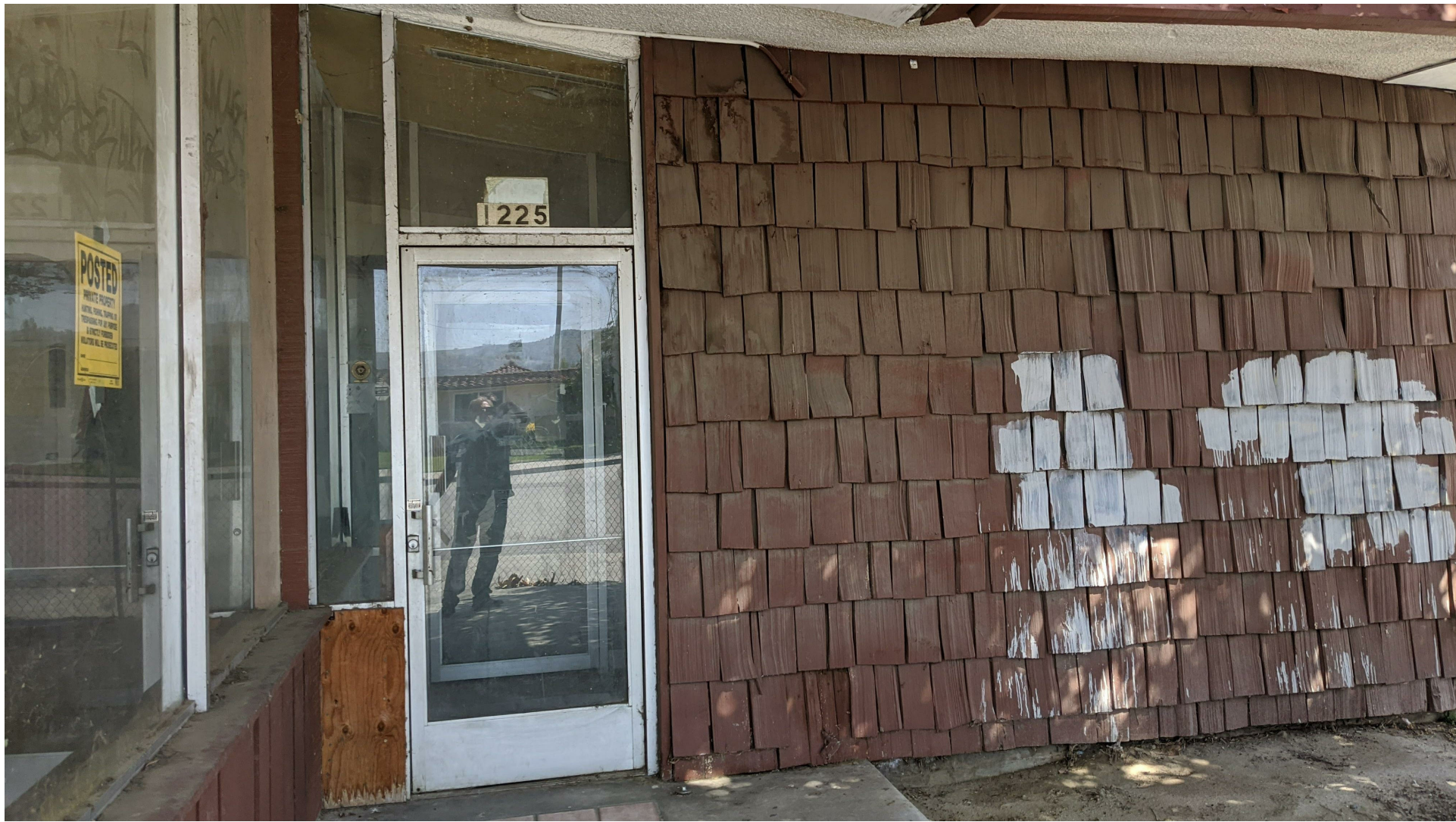
Siding to be Removed
