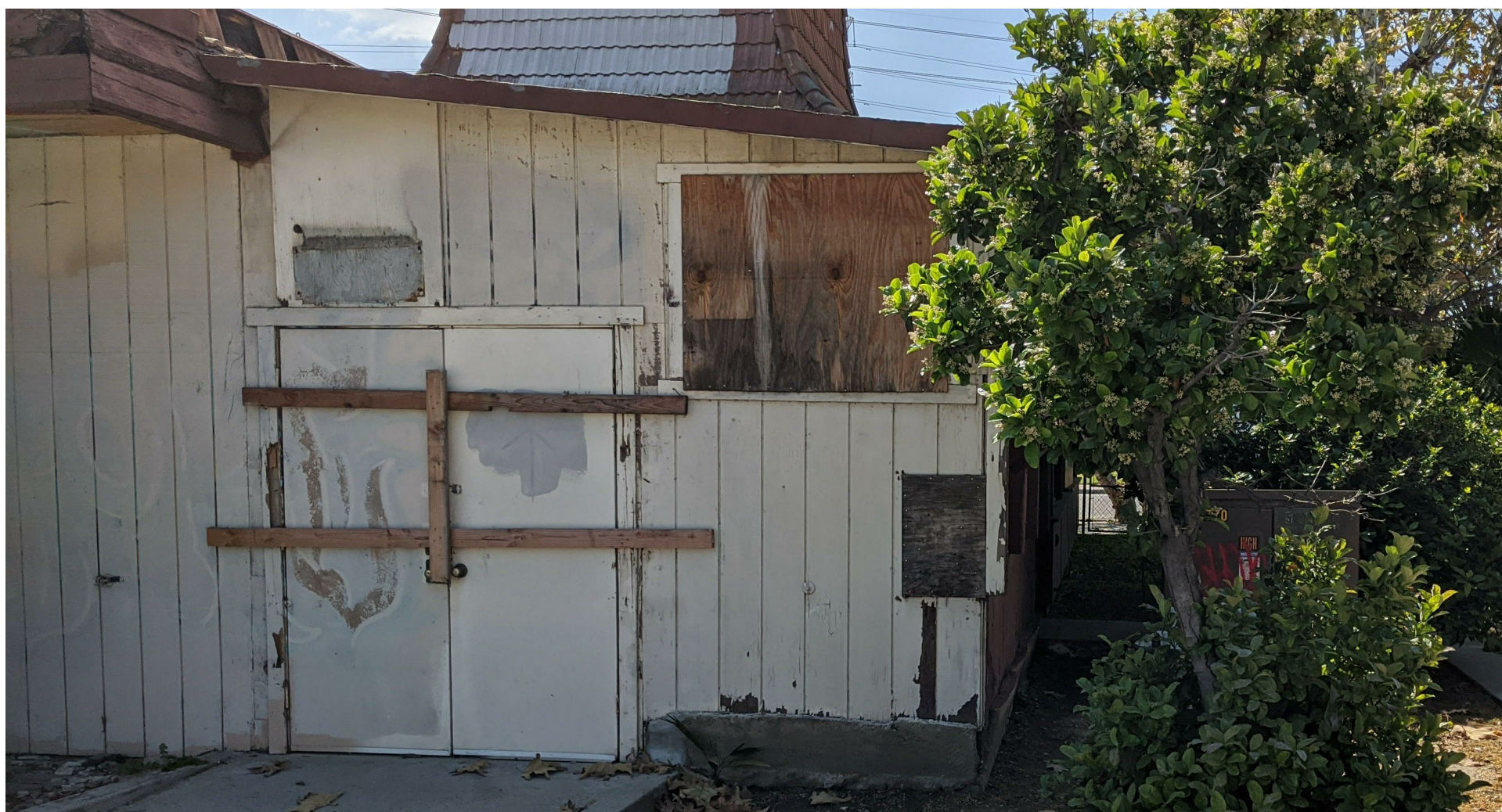
Structure to be Removed
